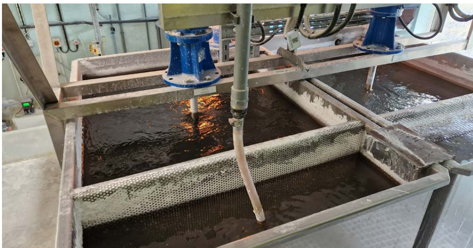
Figure 3.8: pH correction tanks – this reduces acidity and improves water treatment results
